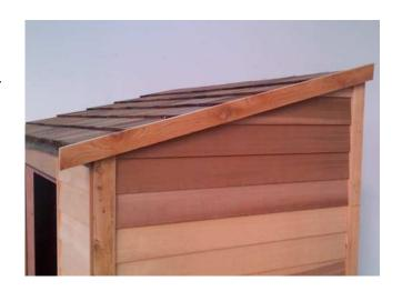
Step 18: Ensure shed is square, by measuring internal diagonals at bottom corner of wall panels.
