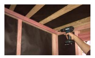
Step 15: Using 2 x 75mm framing nails, nail centre roof support to front and back top plate stiffeners. Predrill if necessary.
