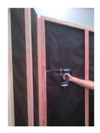
Step 6: Silicone edge of weatherboards on standing panel and nail on cedar beads with 5 x bead nails. (Refer to wall plan for correct beads).
