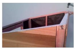
Step 10: Using 30mm Galv Clouts nail top cedar boards to Stiffeners (2-3 per board). Predrill holes to stop boards from splitting.
