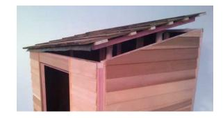
Step 14: Using 75mm tek screws, screw roof panel into end wall panels, (2 screws each end).
